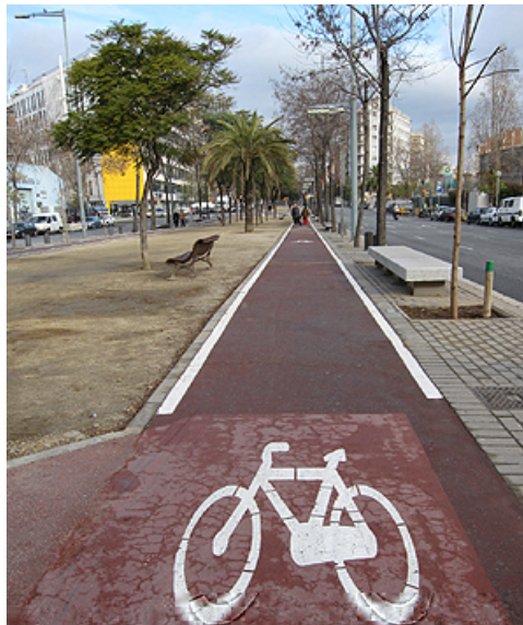
Figure 3.7: One-directional bike lane on sidewalk without any physical separations from other users (“Carril - Bici Av Meridiana (Aragó - pl de les Glòries) | Sant Martí”, n.d.)
