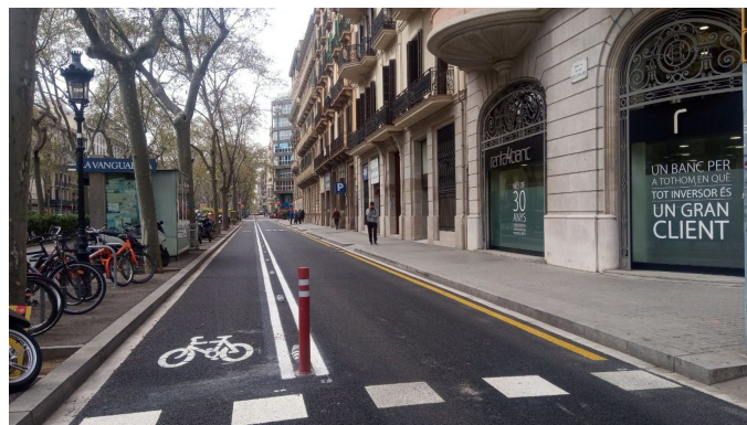
Figure 3.2: One-directional bike lane implemented in the road with low blocks as physical barrier (Pacheco, 2022)
