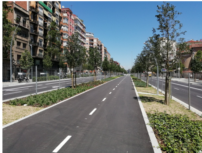
Figure 3.6: Two-directional bike lane in the middle of the avenue, separated by plants and trees from other traffic (Tower, 2019)
