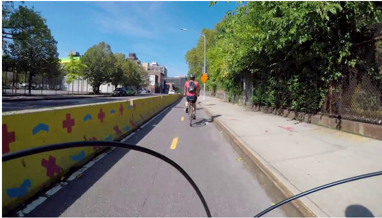
Figure 3.5: Two-directional bike lane implemented in the road, separated with "New Jersey" style blocks (Rozier, 2017)
