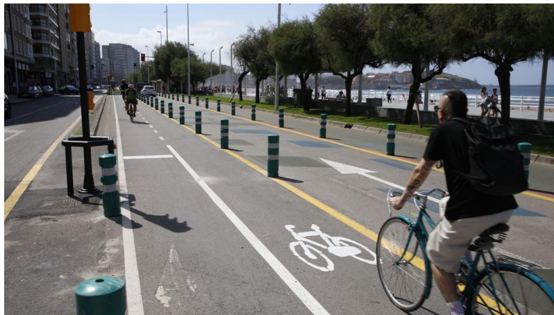
Figure 3.4: Two-way bike lane implemented in the road, separated with cones from other traffic (Puertas, 2022)
