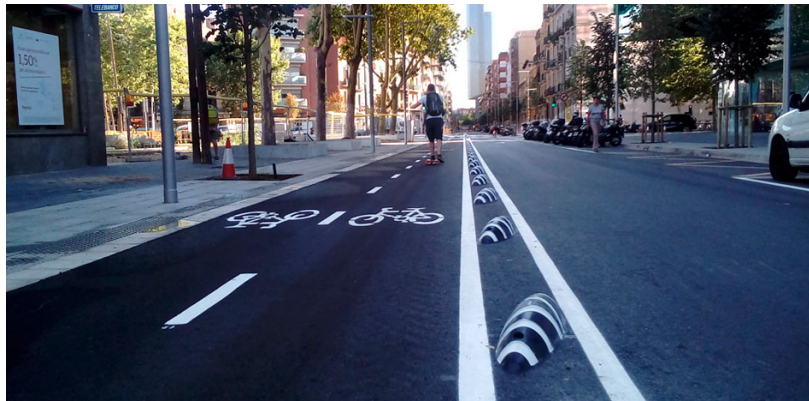
Figure 3.3: Two-directional bike lane implemented in the road with low dense blocks as physical barrier (Campos and Campos, 2023)
